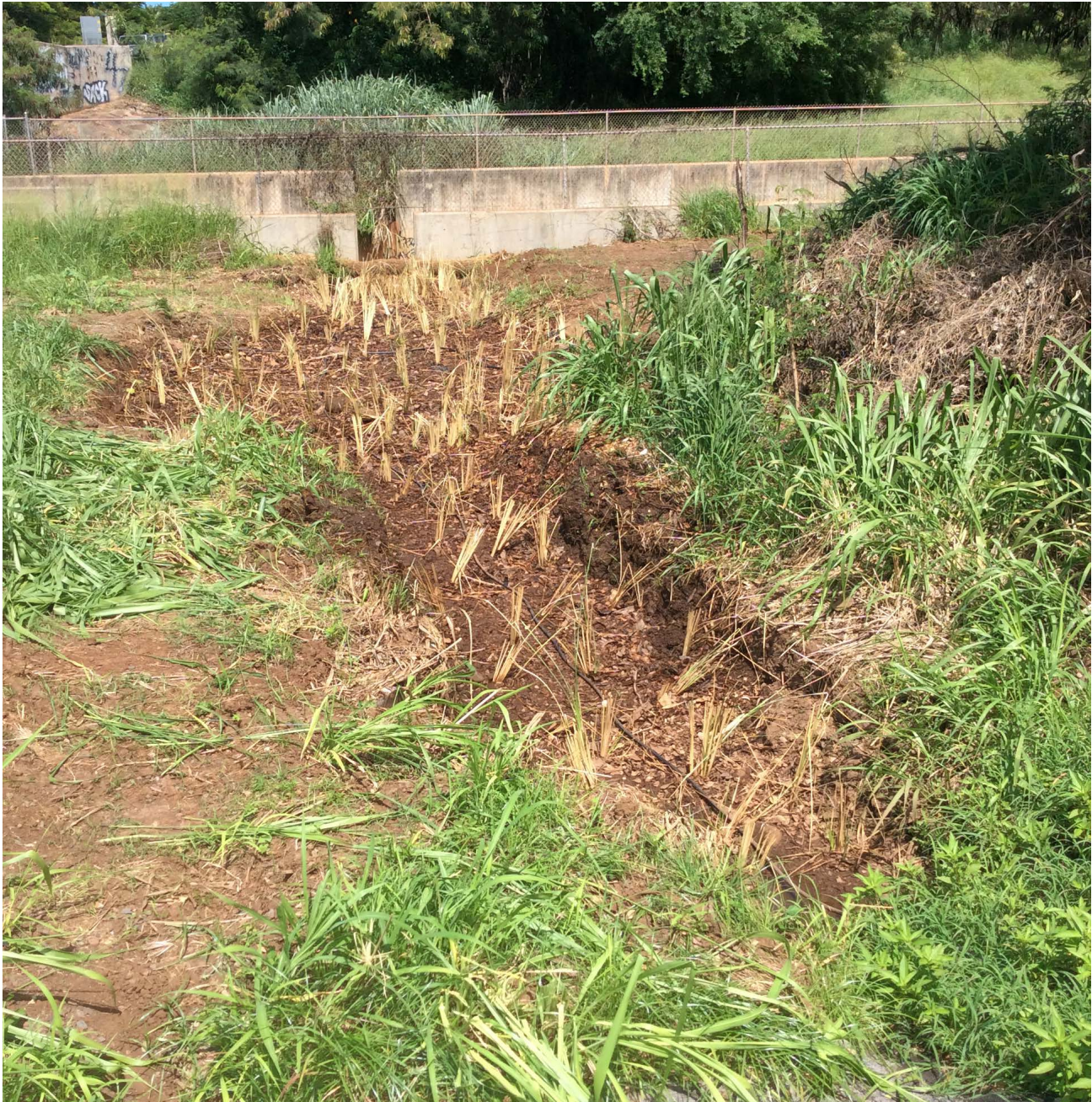
Completed bioretention.
