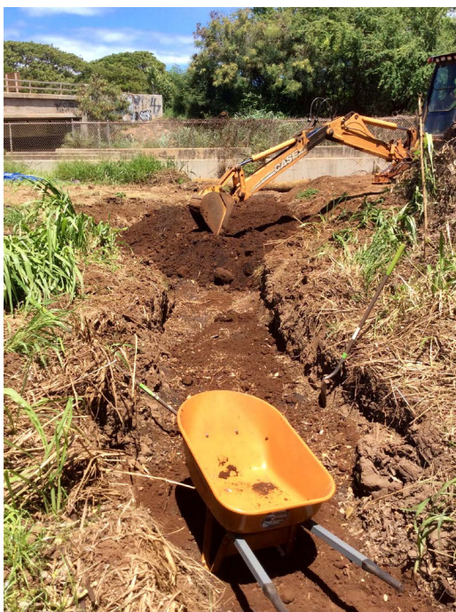
Mechanically sand manually spreading backfill materials.
