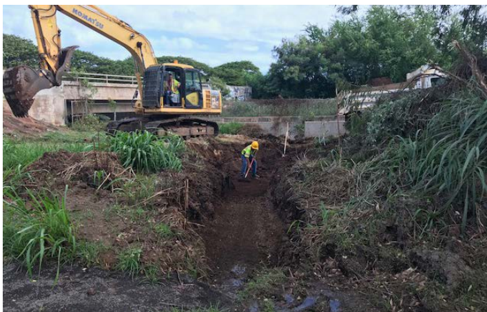
DPW staff excavating the bioretention area.
