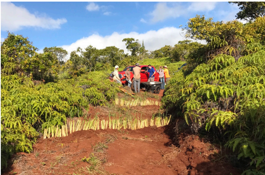
Figure 16. View (from the kickout) of a vetiver sediment trap with adequate vertical storage. (Photo by Paul Sturm)
