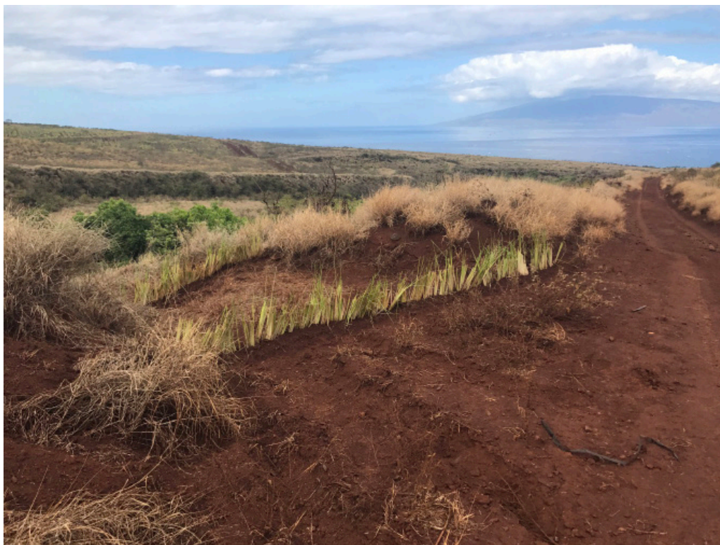
Figure 14. A vetiver sediment trap without proper vertical storage. That is, the first vetiver row is at the same elevation to the road. (Photo by Paul Sturm)
