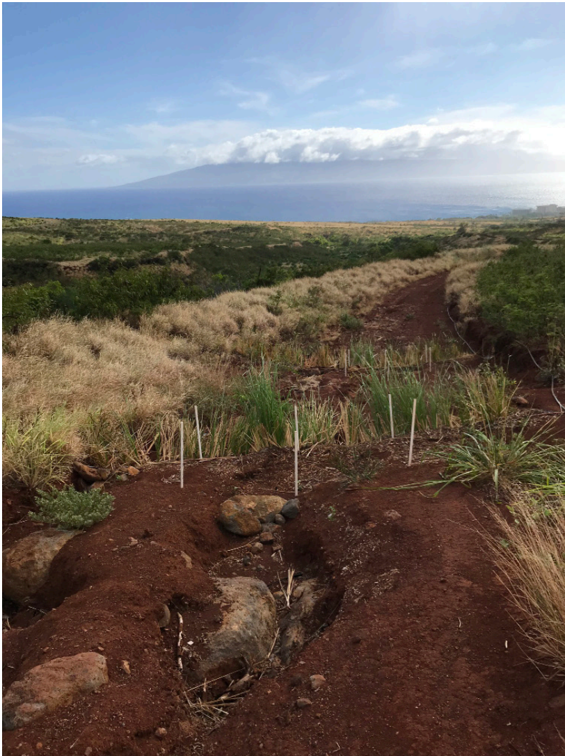
Figure 17. Vetiver sediment traps stationed along a decommissioned road to prevent sediment from being transported down the road. After the sediment has started to accumulate, native plants can be put in to hold remaining soil in place and return the area to its natural ecosystem. (Photo by Jennifer Vander Veur)
