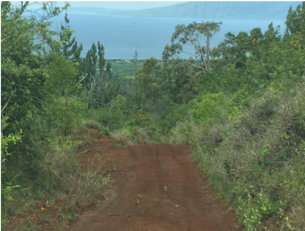
Figure 6. Rolling dip delivering water to a kick out on a dirt road in West Maui. Photo by Paul Sturm
